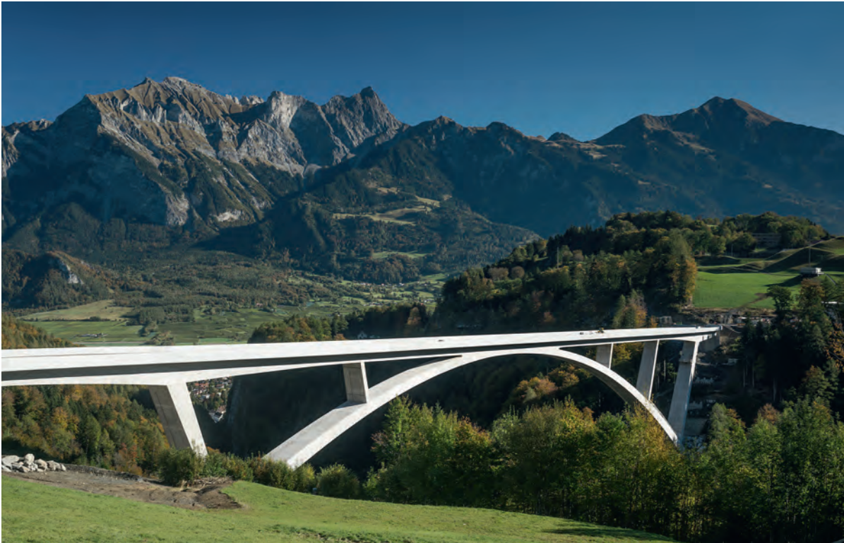
Fig. 9 Die fertige Brücke. The completed bridge. (© Bastian Kratzke)
