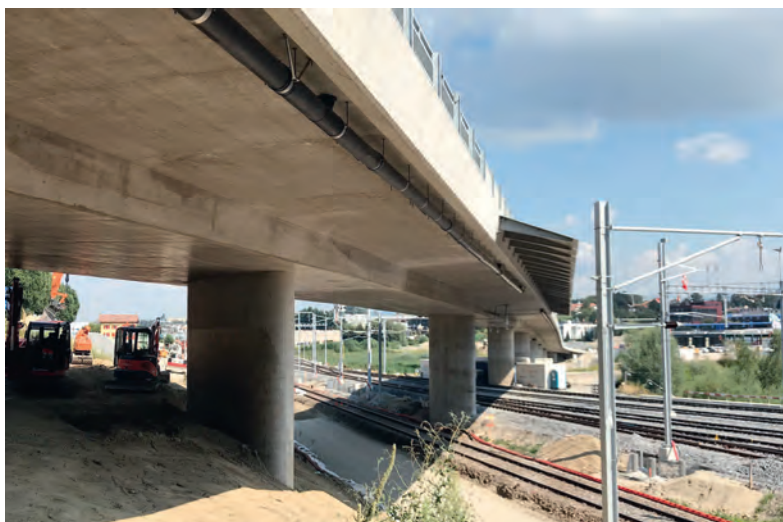
Fig. 2 Vue de la culée nord vers le sud. View from the north abutment towards the south.
