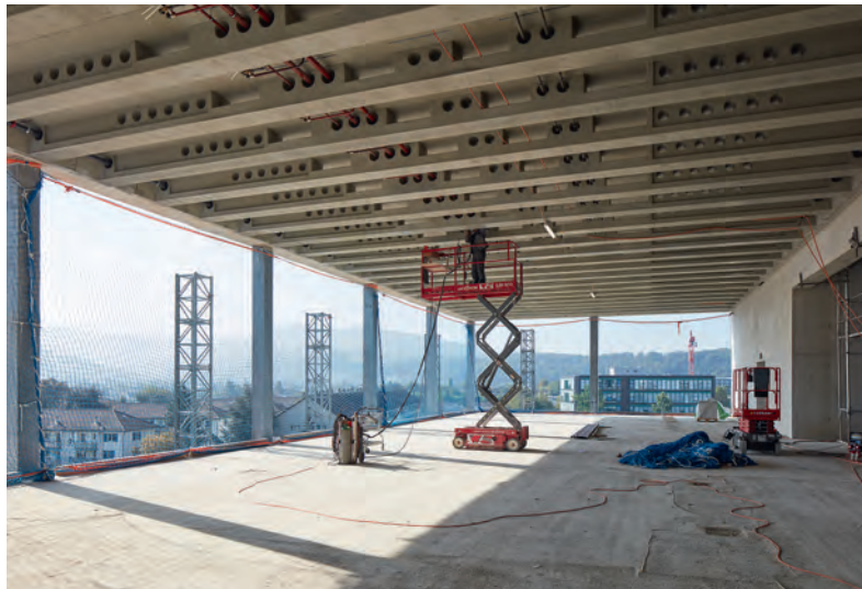
Fig. 6 Fertige Rippendeckenuntersicht. View of finished ribbed slab from below. (© Martin Stollenwerk)
