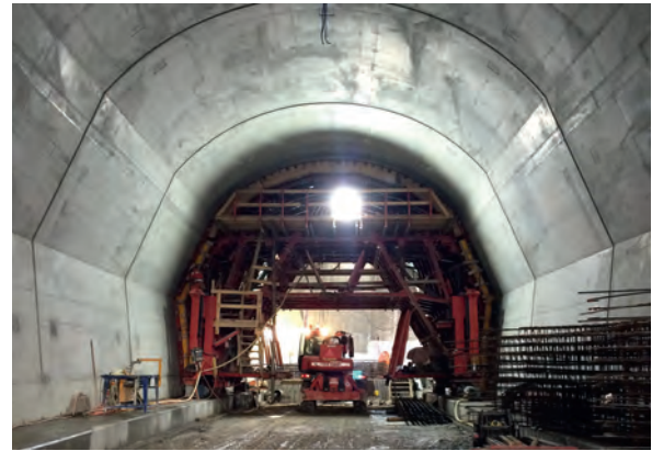
Fig. 5 Vue du tunnel en construction. View of the tunnel under construction.
