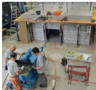
Pre-tensioned double-span slab: injection of tension cables.
