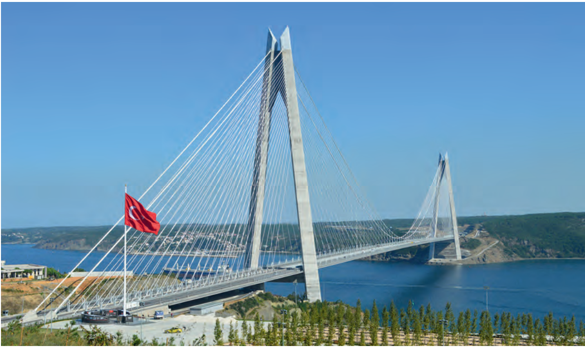
Fig. 4 Forme pure et dynamique des mâts. Dynamic and pure shapes for the tower legs.
