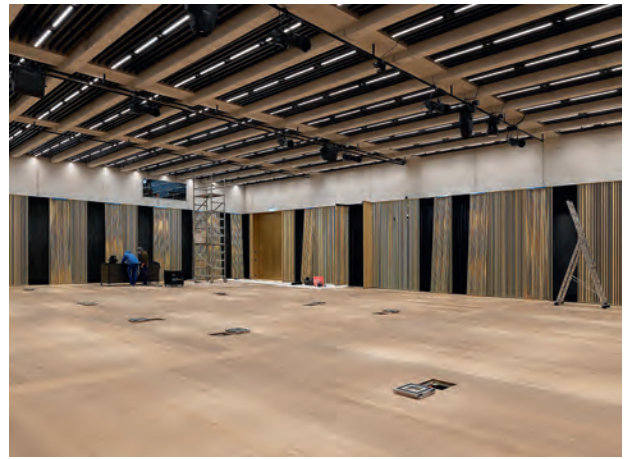
Fig. 4 Festsaal, Deckenrost in Sichtbeton. Banqueting hall, ceiling grid in exposed concrete. (© Beat Bühler)
