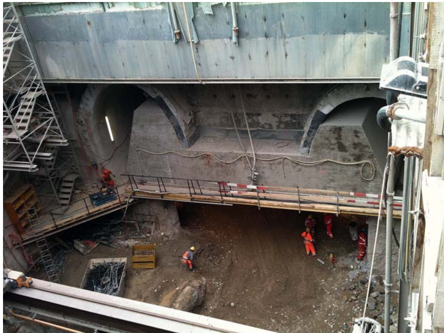
Fig. 8 Aushub unter fertiger Abfangdecke. Excavation work under completed transfer slab.
