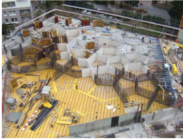
Fig. 3 Die Wabendecke im Bau. The honeycomb ceiling during construction.
