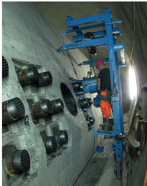
Fig. 7 Hebewagen für Spannprese. Trolley with stressing jack.
